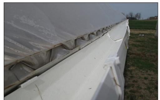
Figure 3: Plastic snap together gutters on a high tunnel. Repair tape was used to fill the gap between the gutter and the structure.
