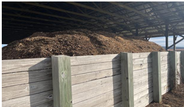
Figure 1. Litter stacked over 7 feet high in a stacking shed. Sidewall is 5 feet high.
