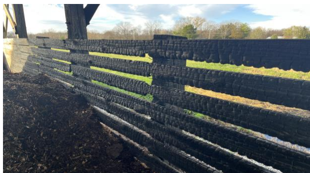
Figure 3. Overheated litter can reach the flashpoint of wood and start a shed fire.
