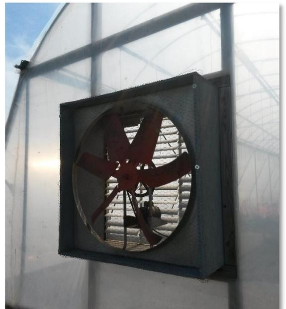
Figure 5. Check the manufacturer's specifications to find out how much air your fan will move.
