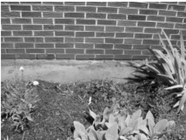
Leave a 12-18 inch bare zone next to the foundation.
